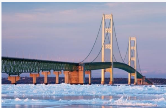
The 5 mile long Mackinac Bridge connects Michigan's upper and lower. It is the longest suspension bridge in the Americas.
